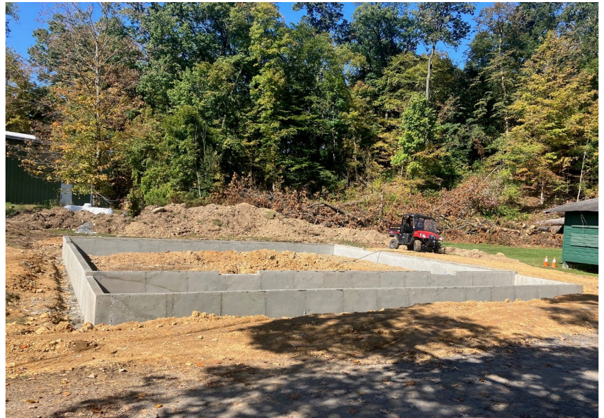
First New Cabin—Pouring the Foundation
