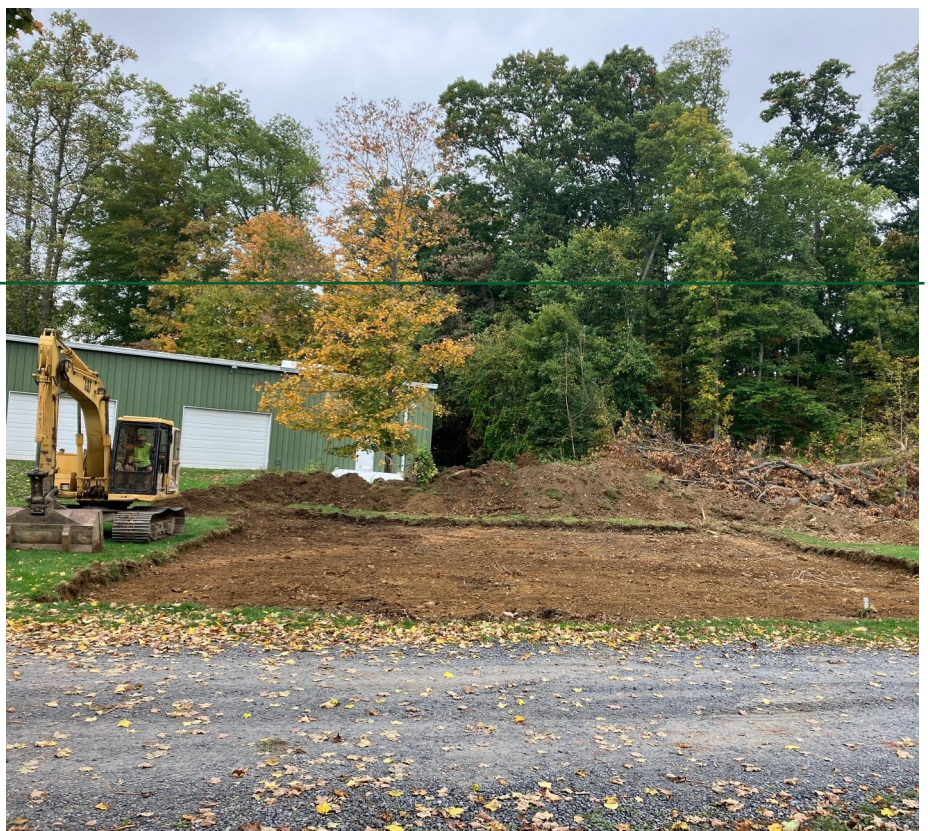
First New Cabin—Groundbreaking and Excavation
